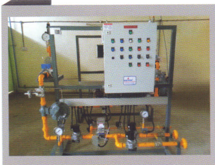
GAS TRAIN WITH CONTROL PANEL
