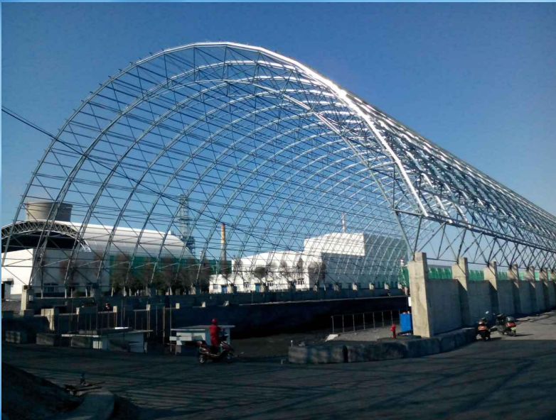
Dry coal shed for CNPC in Dushanzi, Xinjiang (41.5 *100 *20m )
