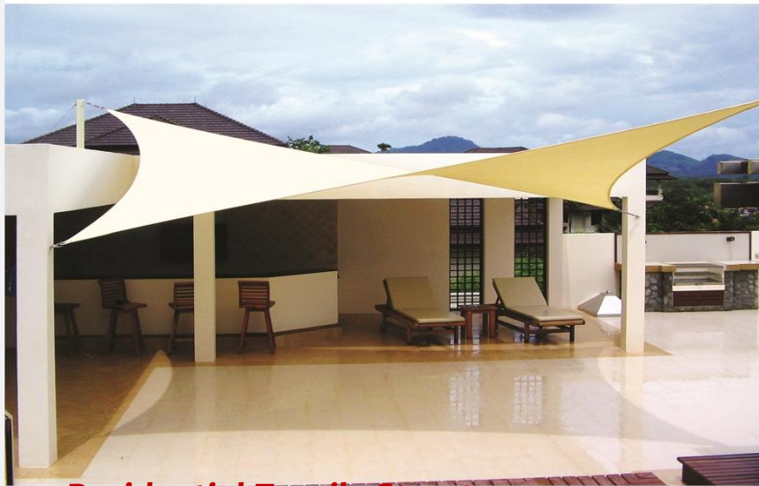
Residential Tensile Structure
