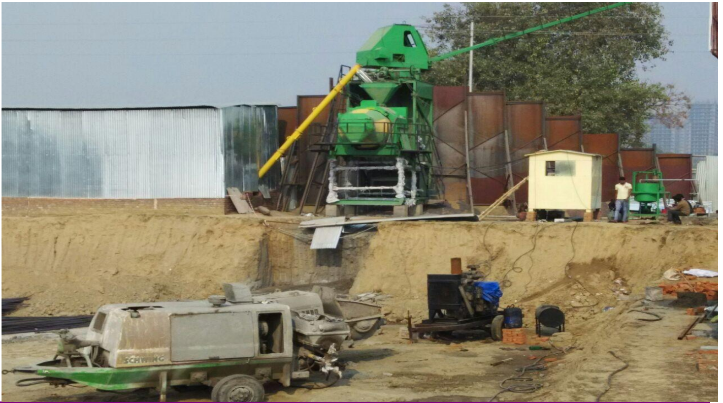
Batching plant machine with pump and Lab testing equipments at Mangalya site>>>
