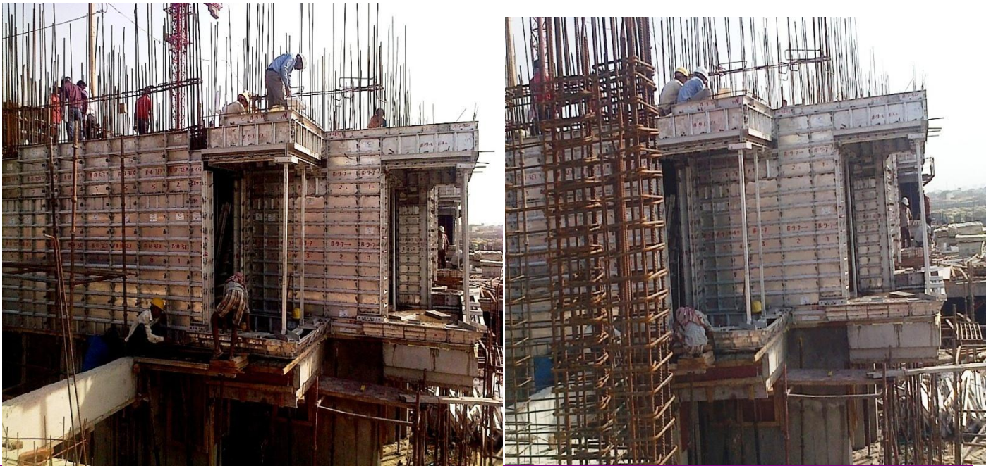
Some photographs of Aluminum Shuttering which is being used in Gaur city Project
