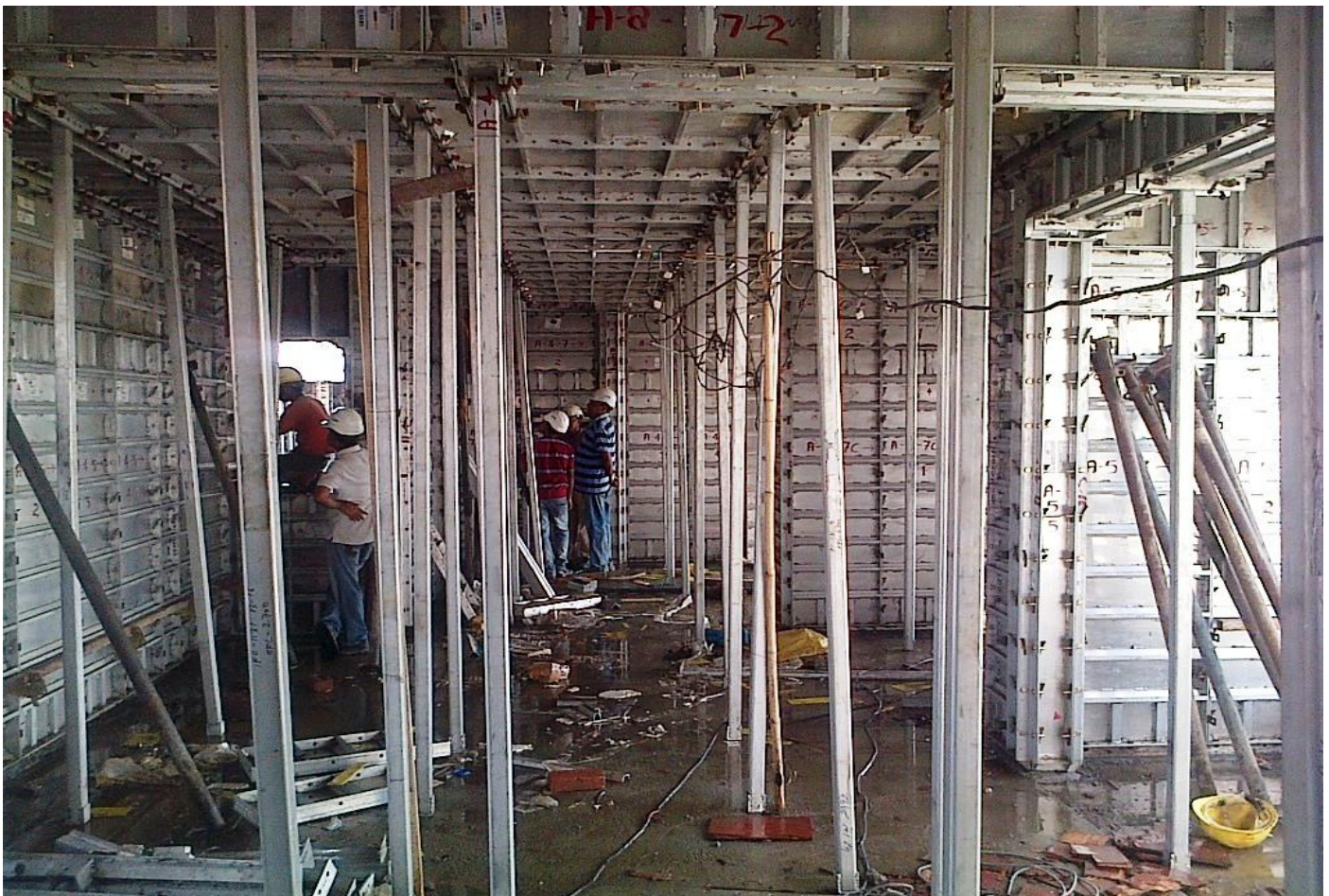
Some photographs of Aluminum Shuttering which is being used in Gaur city Project
