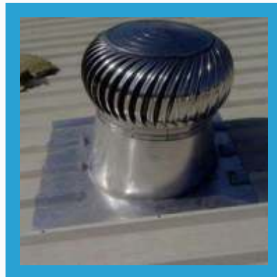
GI Turbine Ventilator
