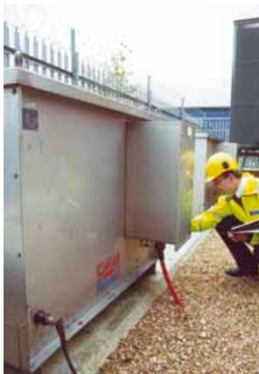
NER rated 11kV, 625A for 10 seconds installed in a substation near Heathrow.
