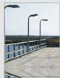
Handrail Mounted Poles For Cooling Towers
