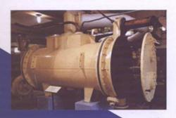
These condensers are heat exchangers which convert steam from its gaseous to its liquid state at a pressure below atmospheric pressure. the purpose of a surface condenser is to condense the exhaust steam and convert the exhaust steam into pure water so that it may be reused in the steam generator or boiler as boiler feed water.
