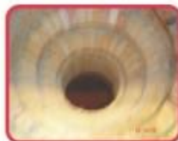
Furnace Brick Work At Coil Bottom
