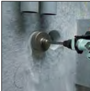
TCT core drilling
