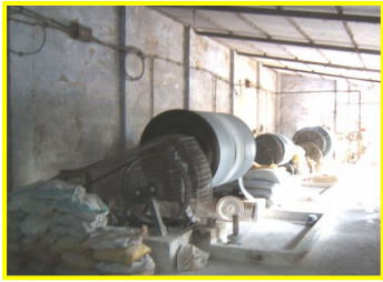
Raw material milling & mixing
