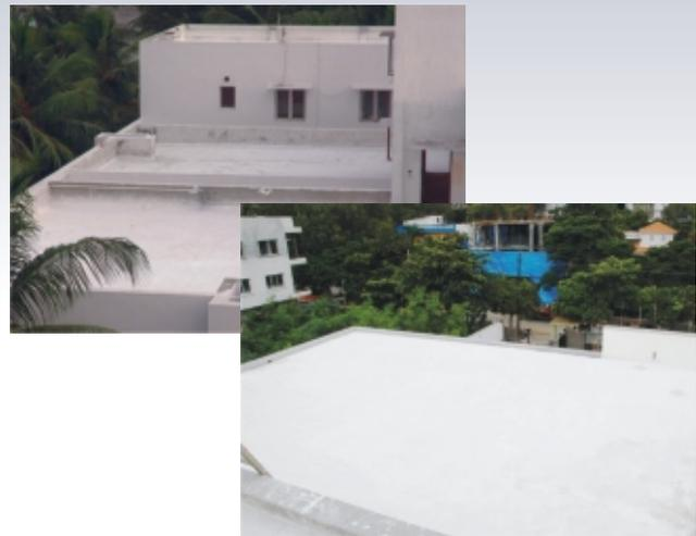
THERMATEK® Heat Reflective Paint is designed to combat overheating in metal or asbestos or flat roof buildings.
