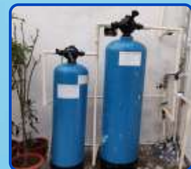
Sand Filter + Water Softener
