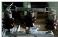
11 Kv Rotating Isolator
