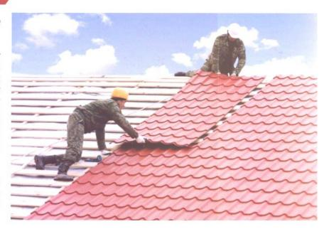
The roof truss structure adopts sectional steel purlin, the purlin is required to be flat without deformation, and two purlins must be in the parallel with uniform span of 700mm.
